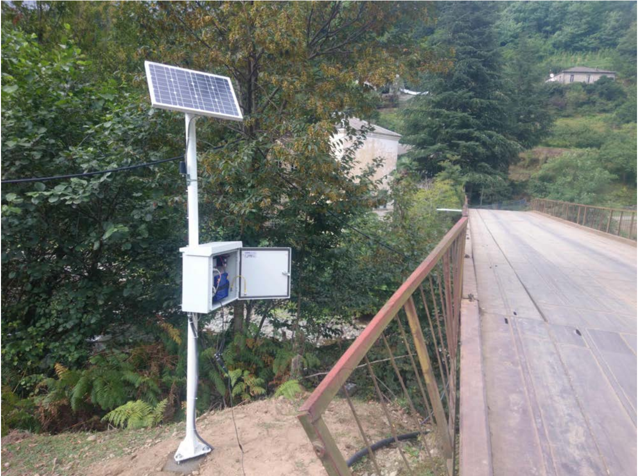
Figure 6: Datalogger General View
