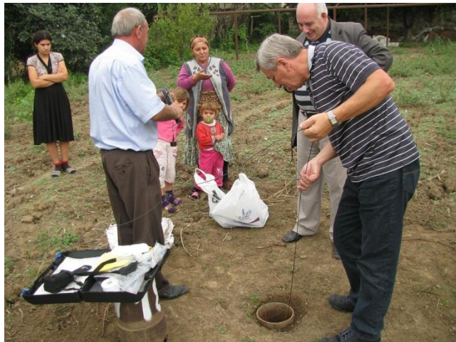
Installation of water level meter in the monitoring well
