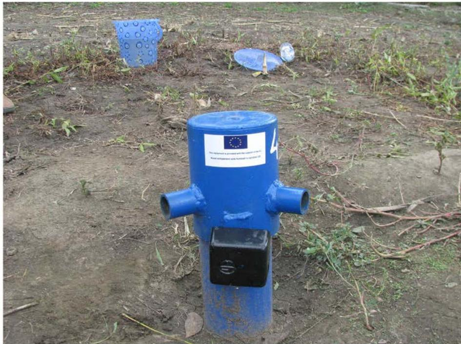
Figure 1. Refurbished borehole with protection wellhead
